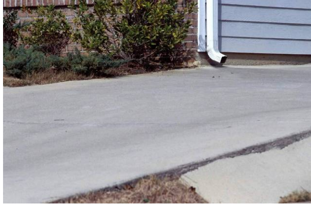
A directly connected roof drain
