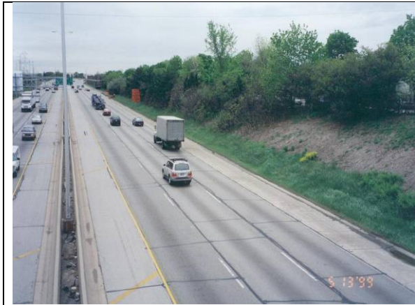
Depressed downtown freeway with eroding embankment
