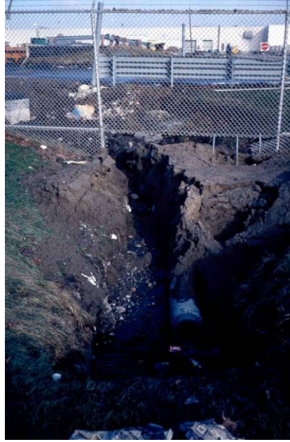
Scoured drain from paved area.
